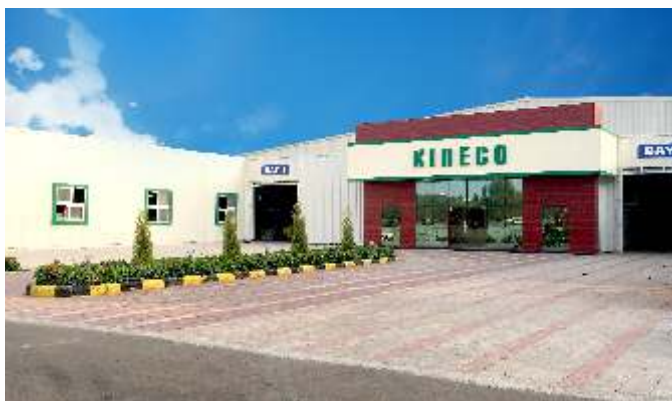
Kineco Railway Unit
